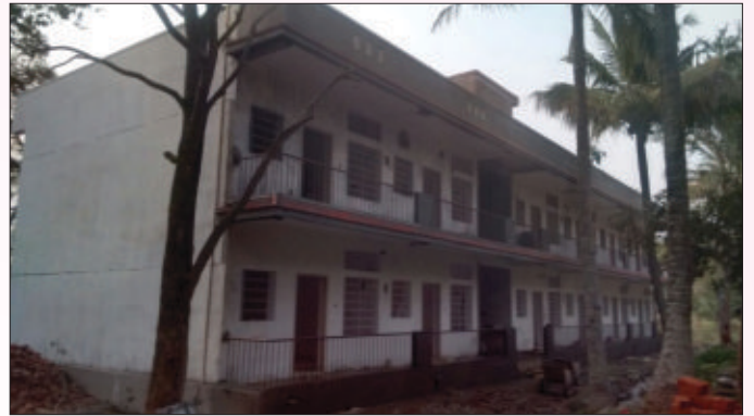
Block A nearing completion –15th Dec.2014
